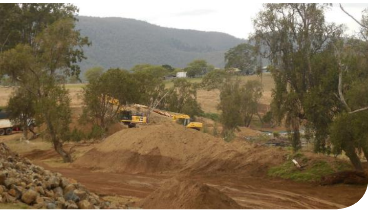
Early construction stage of the project
