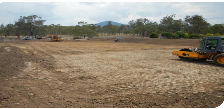
Early construction on the Aratula STP
